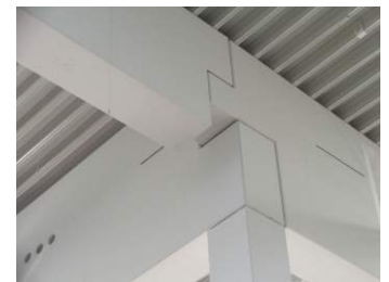
Bearing knot of three pretensioned concrete truss
