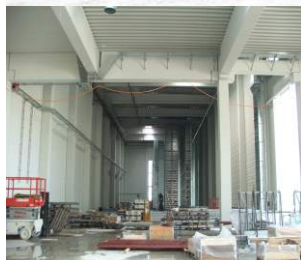
Automated small-parts warehouse
