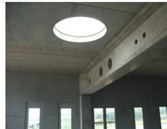
Ceiling with openings for light domes
