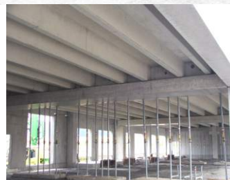
Pretensioned p-slab ceiling on joists with a span of ca. 17 m
