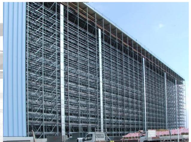
View longside of high bay warehouse, height ca. 35 m
