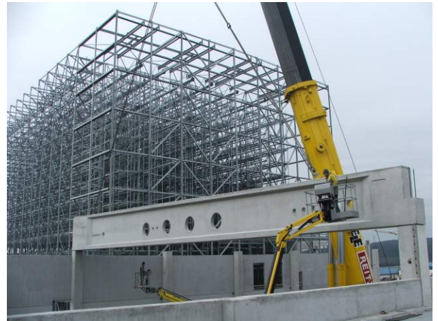
Truss installation, high rise rack in the background
